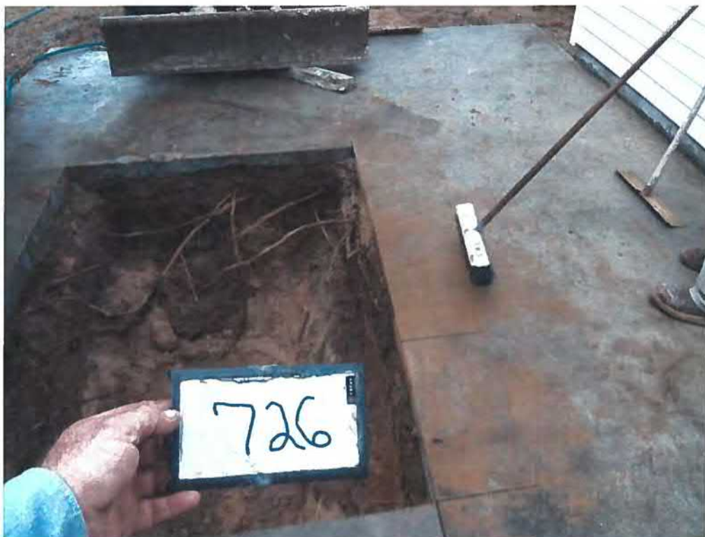
Picture 2: UST 726Bluebell excavation.
